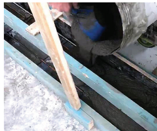
Pouring the Emer-Patch Horizontal Quick Set
